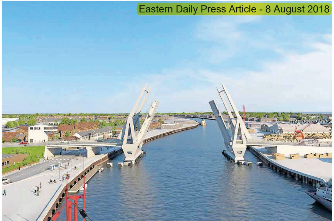
Illustrative design to show one of the opening mechanisms being considered for the third river crossing in Great Yarmouth
